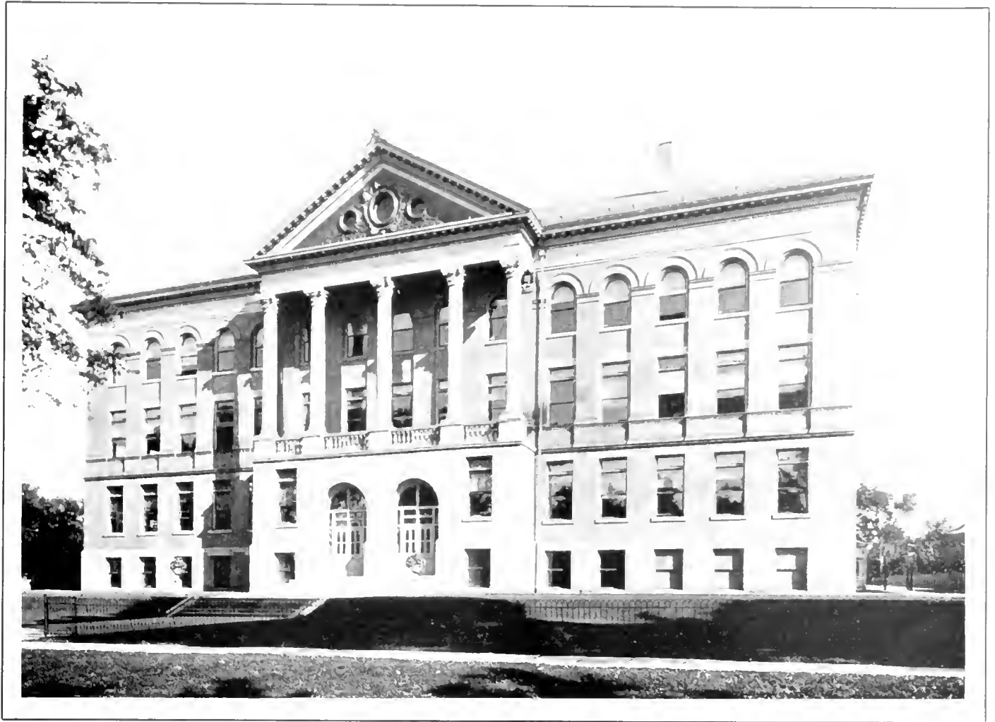
ULICA FREE ACADEMY — KEMBLE STREET Completed 1866, at a cost of $135,000 — The building is 140 x 181 feet, and has capacity for 800 pupils
